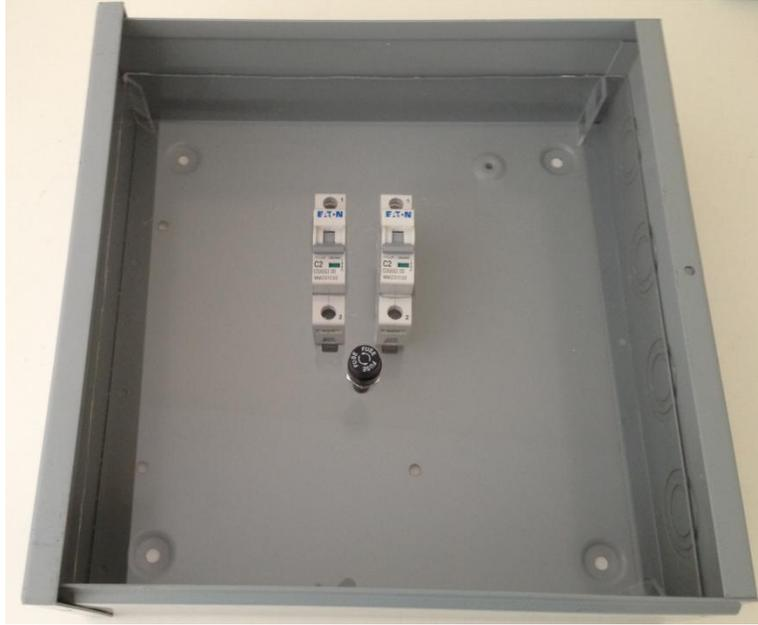
**Figure 3-6: Final Layout in Distribution Panel with Components**
