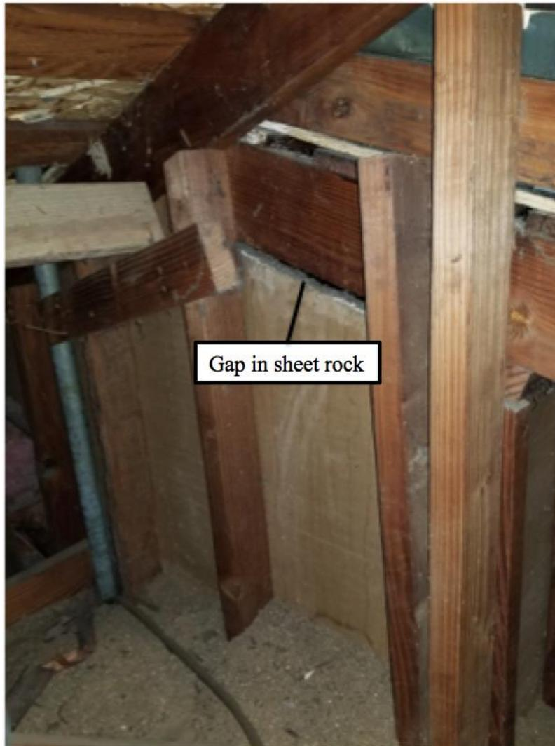
*Figure 7. Framing of existing home to garage addition*
