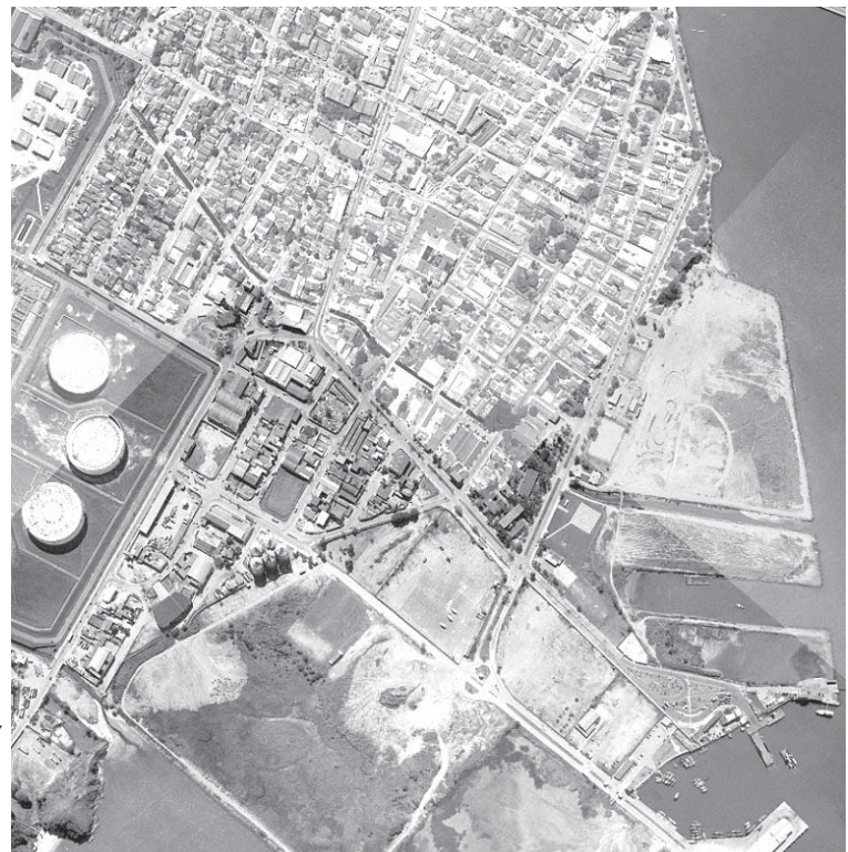
Figure 3. Vila Amelia, an illegal settlement dangerously next to oil containers.
