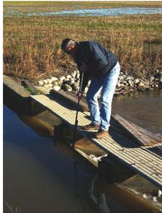
Figure 3. Using the ITRC Weir Stick to pull boards
