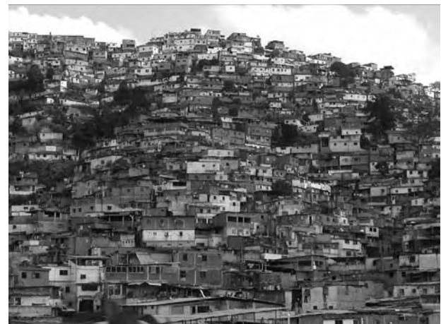
Figure 6. The high density unplanned development of a Caracas Barrio (Photo by W. Siembieda)
