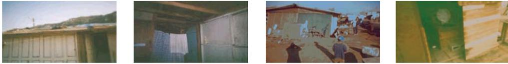
Figure 23: House Constructed of Second-Hand Salvaged Doors
