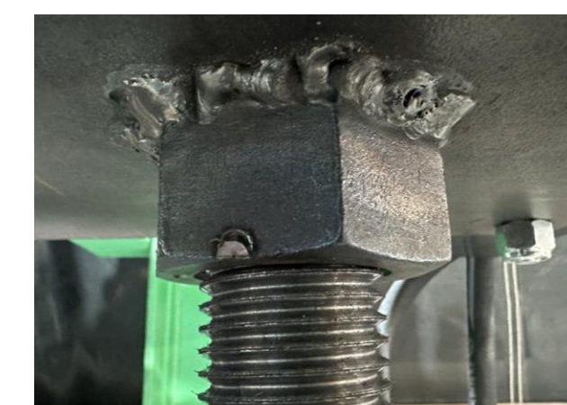
Weld - Nuts for Threaded Rod
