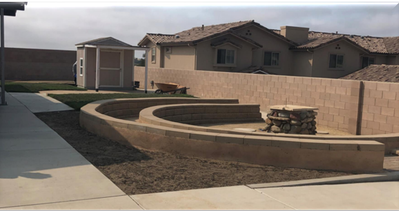
Proposed location for the Veterans Memorial Wall to be mounted on existing CMU wall and be incorporated near the existing sundial seating area.
