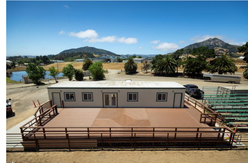
Completed Deck at Cal Poly Rodeo arena
