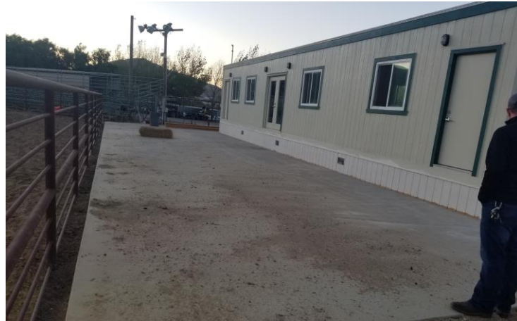
Original slab at Cal Poly Rodeo arena
