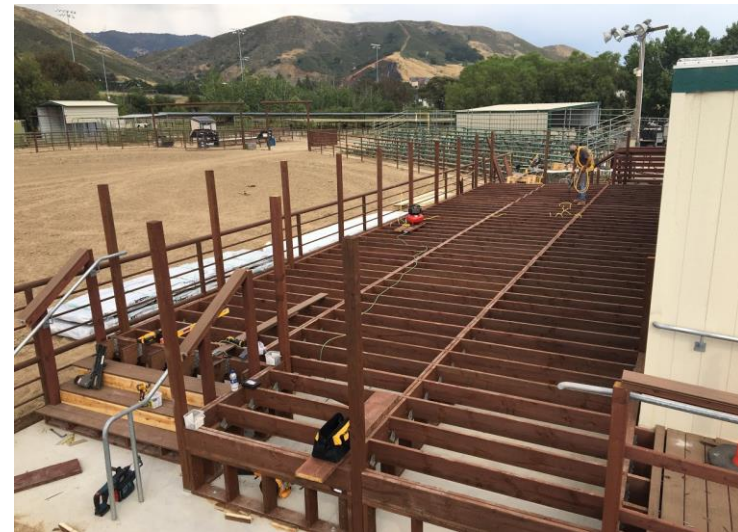
Completing joists and blocking at rodeo observation deck
