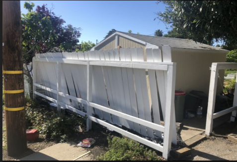
Painting Pickets before securing to rails and posts
