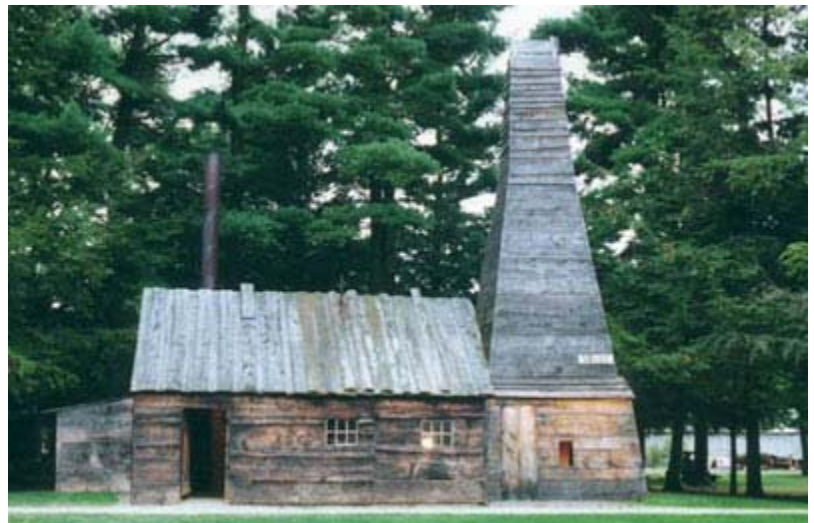
Working replica of original Drake Well. (Photo credit: The Drake Well Museum)
