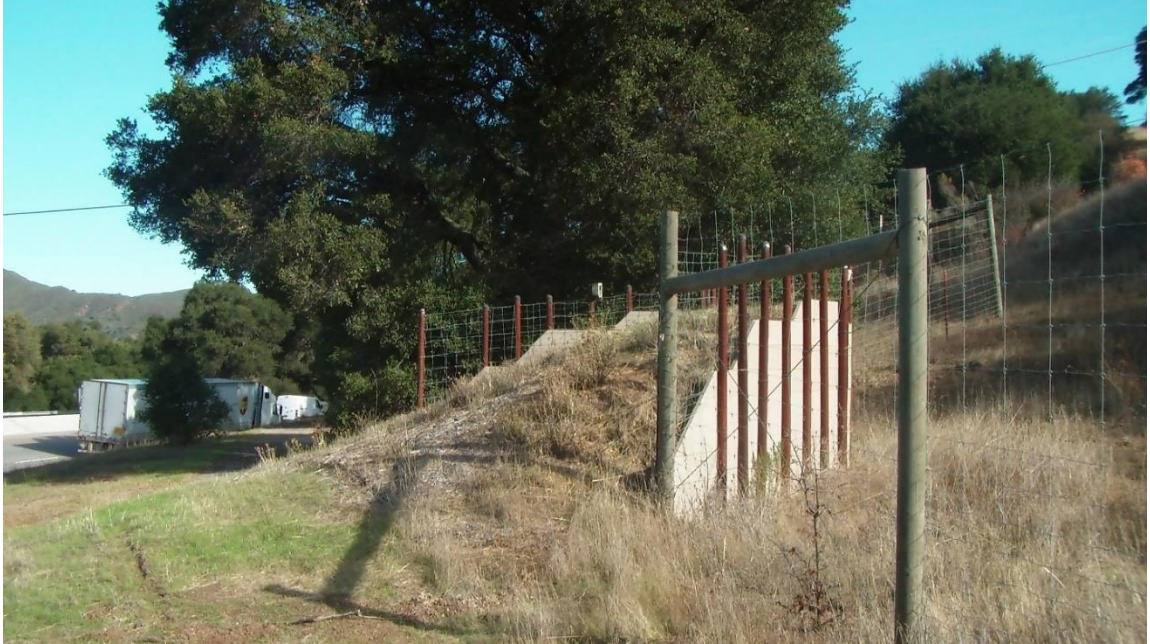
Figure 2.1: Jumpout ramp along Highway 101 in San Luis Obispo County, California (TjCk-N site).
