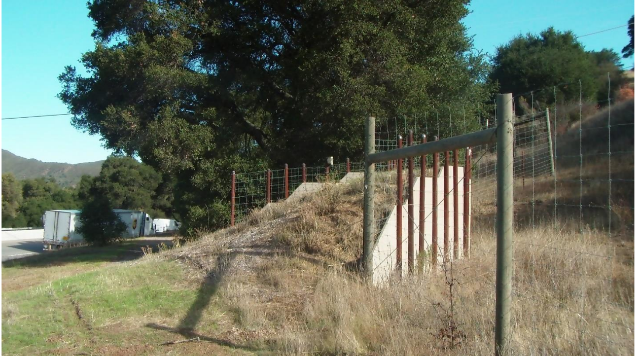
Figure 1.1: Jumpout ramp along Highway 101 in San Luis Obispo County, California (TjCk-N site).
