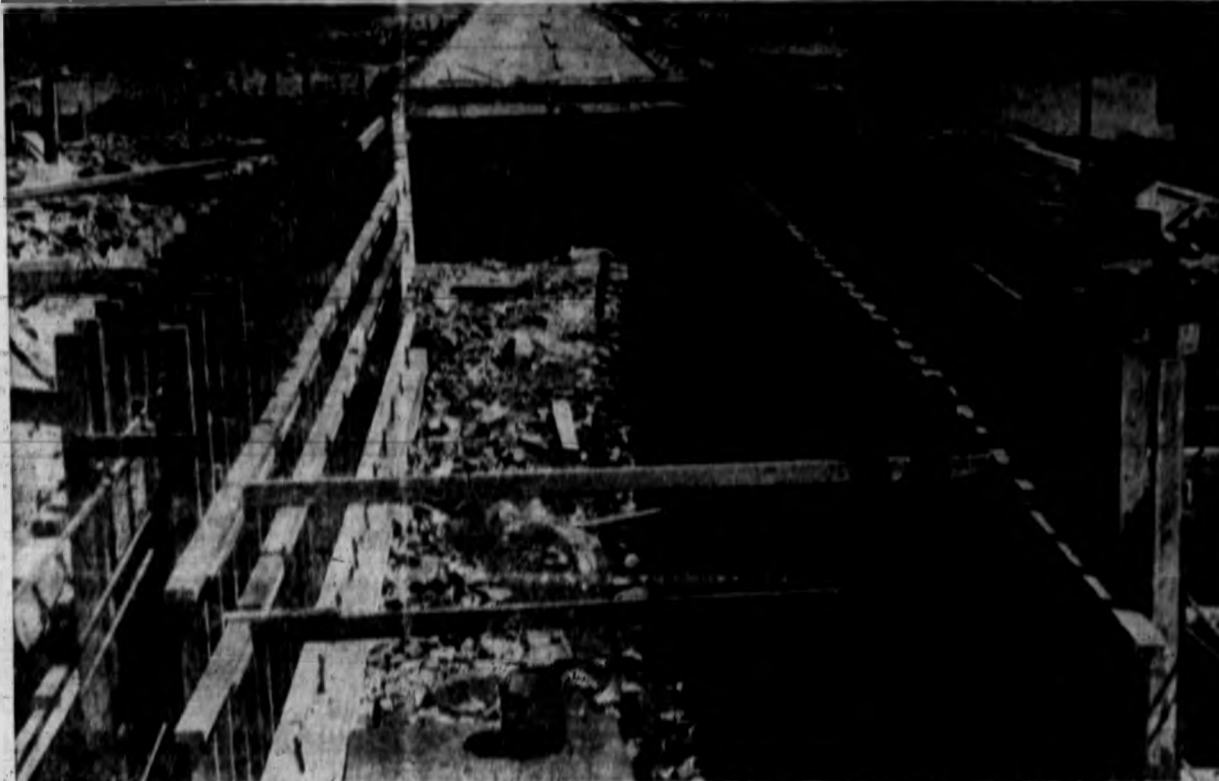
WHAT GIVES! Is it a bomb shelter? Maybe a subway? Or perhaps an underground strategic headquarters for deep dark plots? Nope—only the new conduit chambers under the rising wing of the Engineering building. It's part of the master plan—will carry steam pipes and other utilities across campus under the building.
