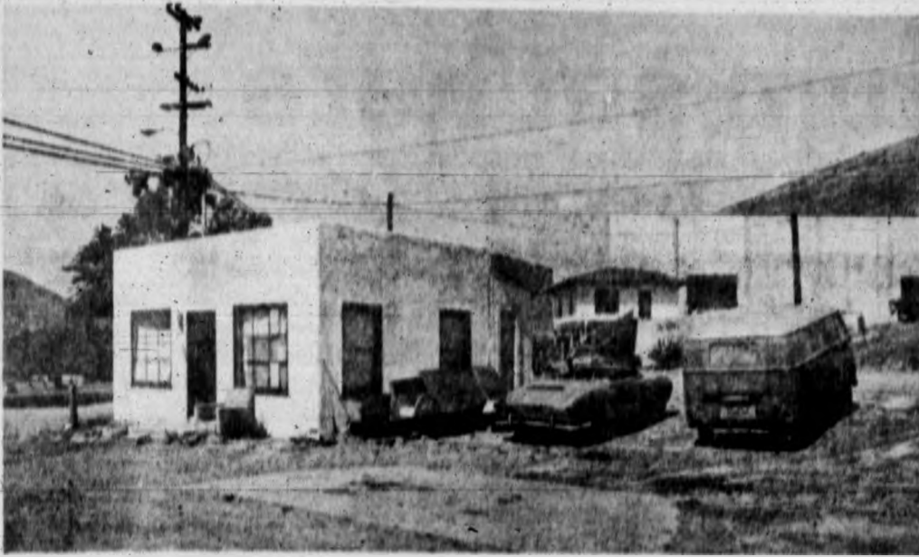
This humble abode used to be "home" for two of the caretakers for the warehouse behind Tiki Tom's Things on lower Higuera. Photo by Barney Guzenke
