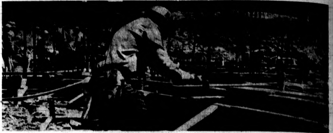
WORKERS START... laying the foundation for the Julian A. McPhee College Union Building. The structure is expected to be completed by October 1969. (Photo by Olson)
