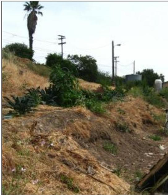
**Figure 5: A terrace with insufficient vegetation**
