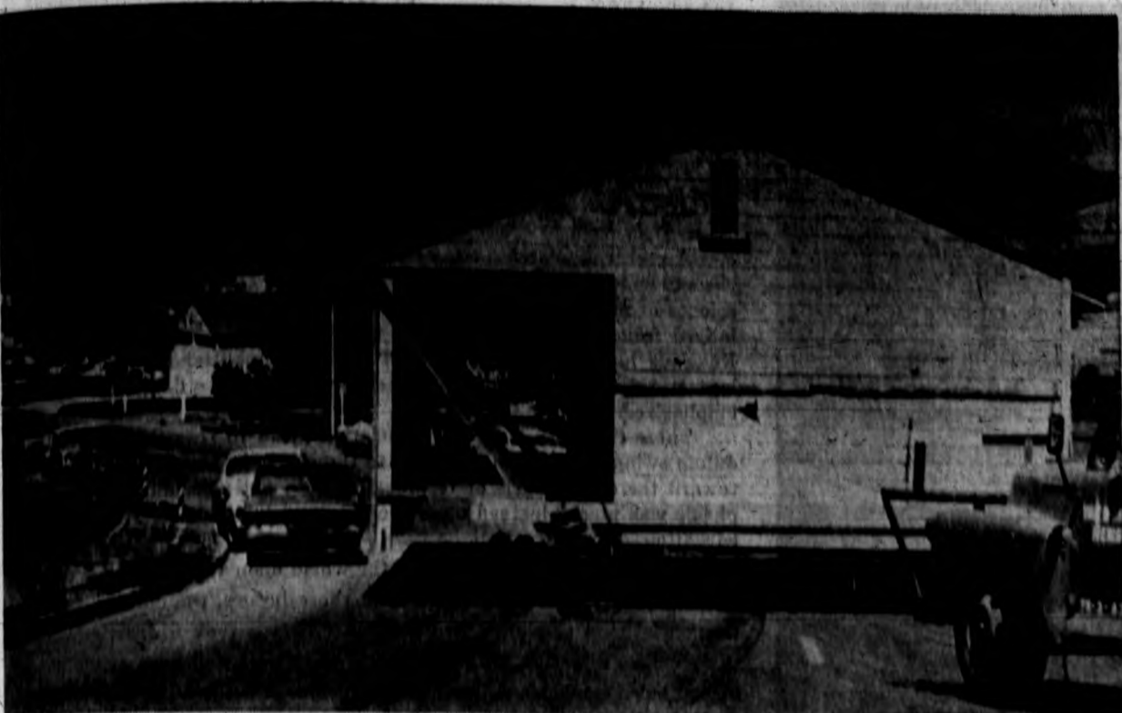
ON THE MOVE . . . A portion of the horse barn previously located at the Thoroughbred Unit is being moved down North Perimeter Road on its way to a new location at the north end of Pepper Lane. The move is being made to make room for a new Corporation Yard. Work on the Corporation Yard has started—a $100,000 project.
