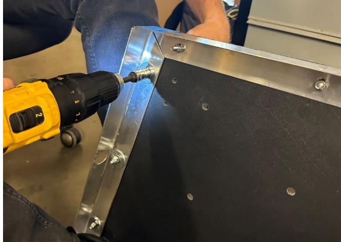
Figure 73 – Group member using drill with socket attachment and Phillips head screwdriver to tighten bolts into place.
