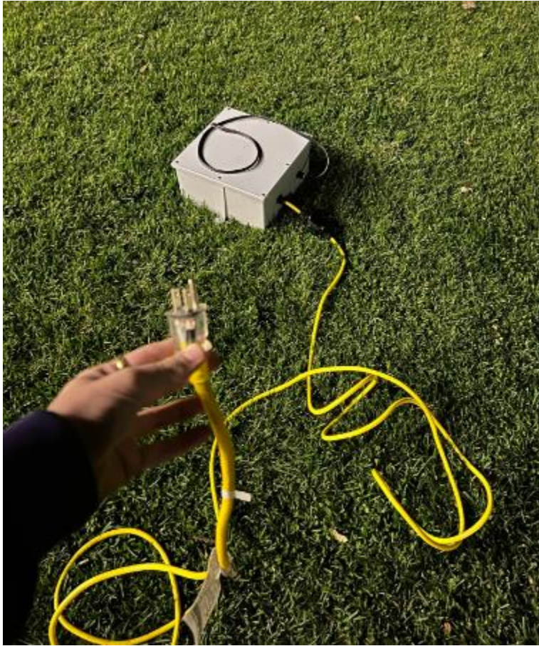
Figure 117 – Power supply near projected start of path. Plug in the end of the yellow cable to a wall outlet.
