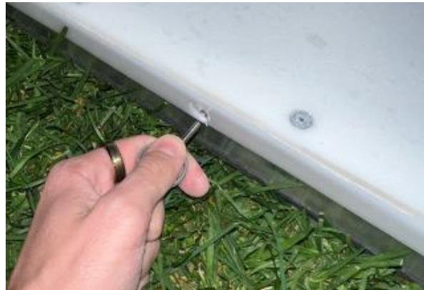
Figure 137 – Reinserting the quick-release pins. Make sure the pin goes through both the white top panel and metal hole. Ensure all 3 are replaced on every tile.
