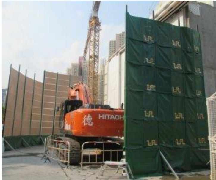
Figure 2. Sound Barriers Source: (Construction Noise Barrier, n.d.)
