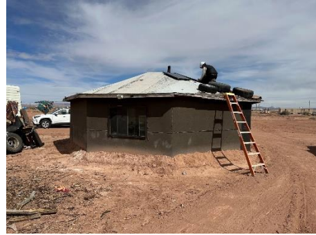
Figure 2. Navajo home undergoing installation
