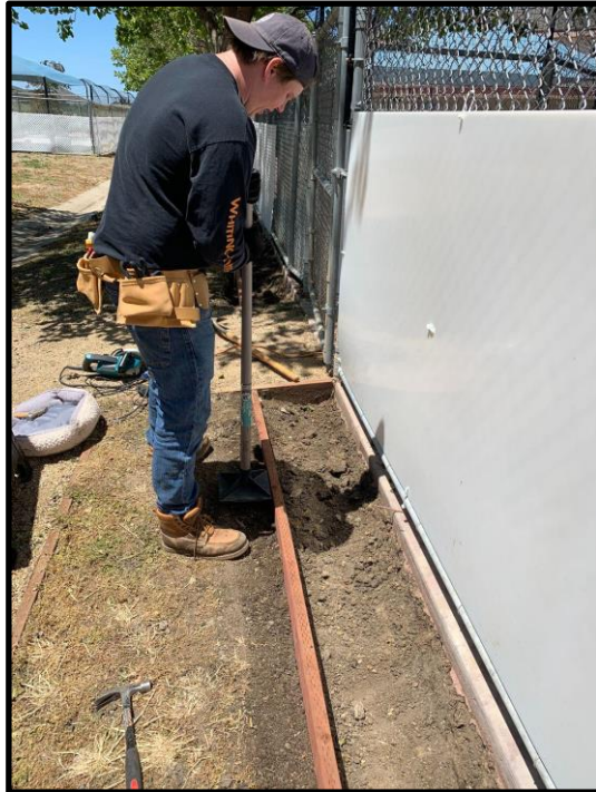
Figure 7 - Tamping the Backfill
