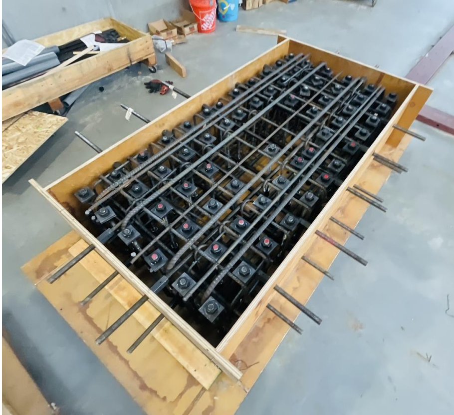
Figure 2. Rebar Cage and All-Thread Top View.
