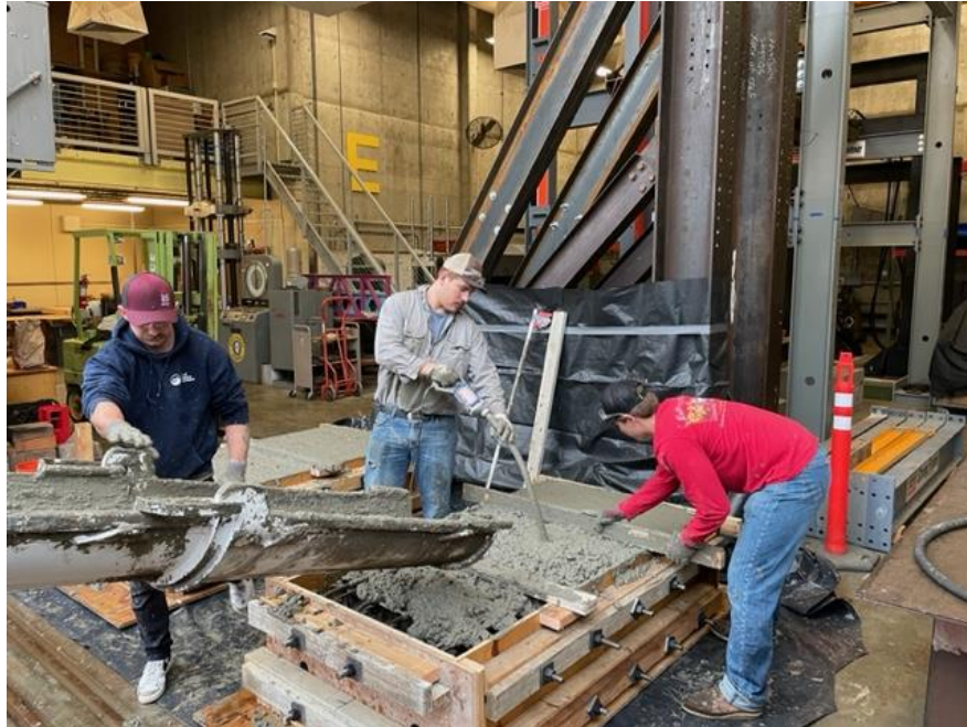
Figure 6. David, Henry, and Blaize pouring the footings.
