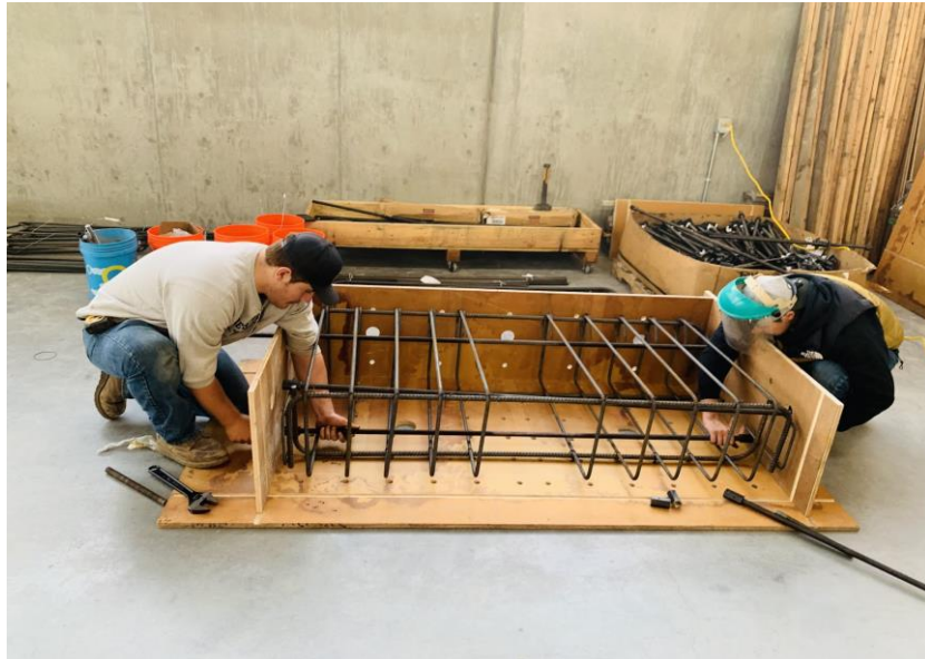
Figure 4. Henry and Blaize tying the rebar cage.
