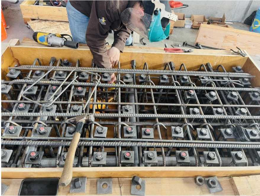
Figure 5. Blaize trimming the conflicting rebar cage to slide PVC in place.
