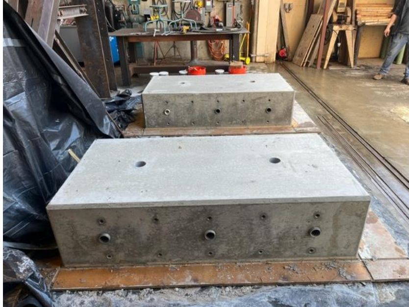
Figure 7. The finished product, both footings stripped with chamfer details.
