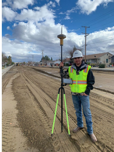
Figure 1- GPS rover and data collector at work in Avenal, CA
