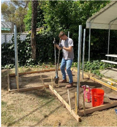
Figure 4. Setting posts prior to pour
