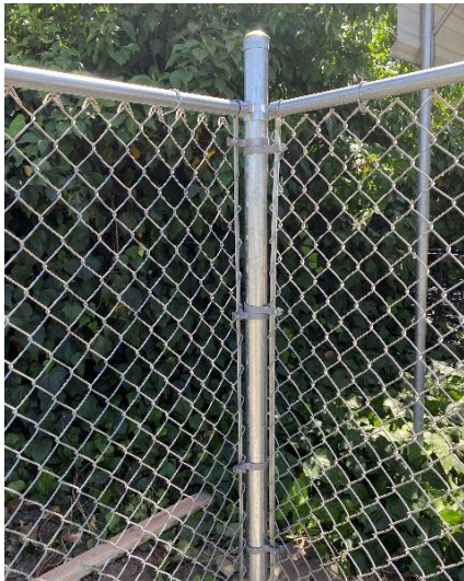
Figure 6. Finished corner with tension bars, tension bands, and metal ties.
