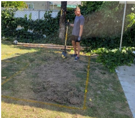
Figure 2. Spray painted border for excavation Figure 3. Completed Excavation after day 1
