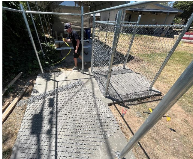
Figure 7. Measuring the chain link section before hanging
