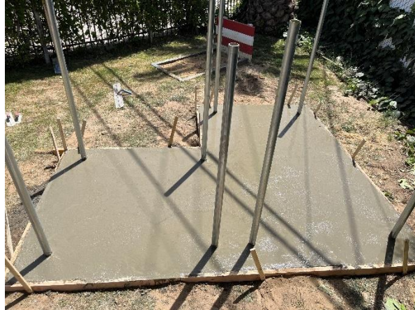
Figure 5. Finished concrete pad directly after pour
