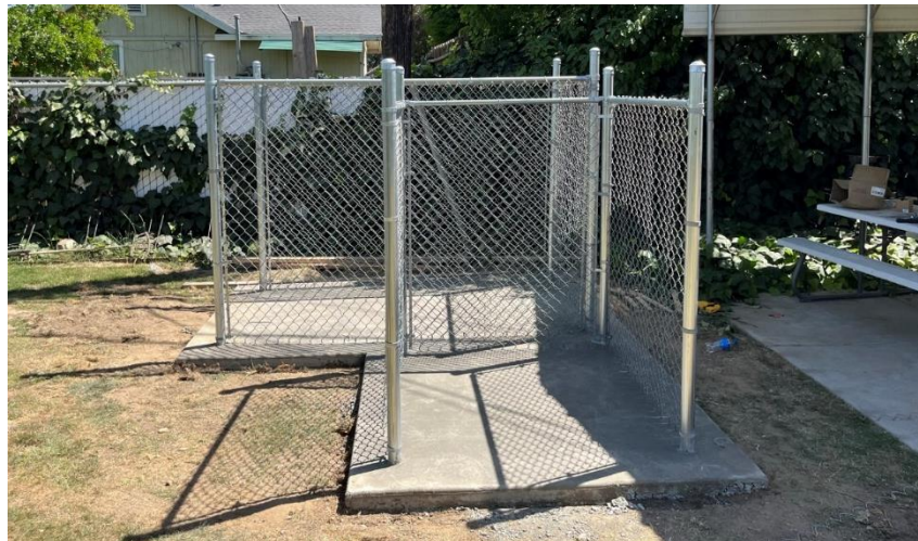
Figure 8. Finished kennel structure before gate instillation
