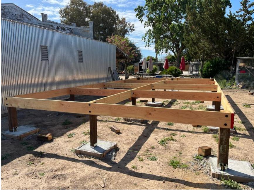
Figure 3. Tall Deck Primary Beams
