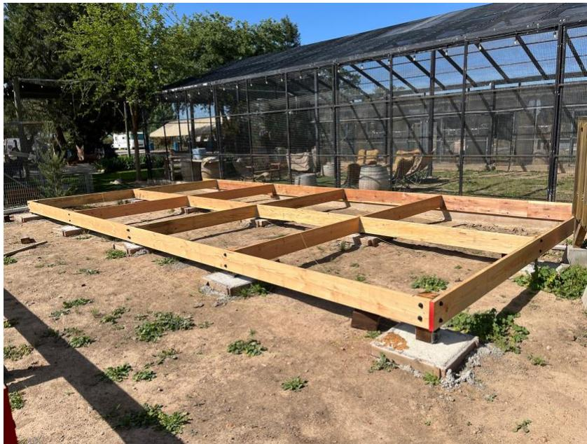
Figure 2. Short Deck Primary Beams
