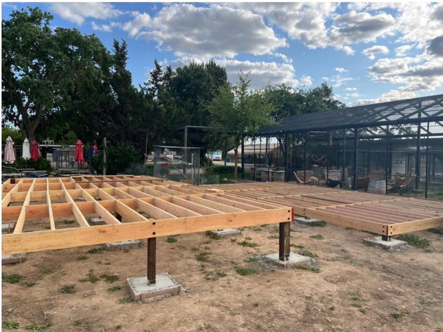
Figure 4. Secondary Member Joists
