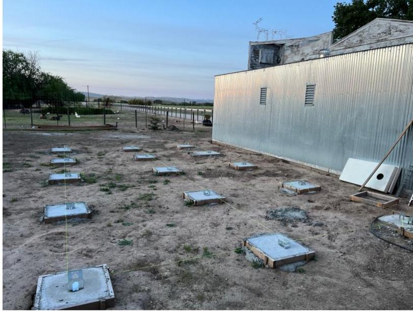
Figure 1. Concrete Footings, Formwork, and Post Bases
