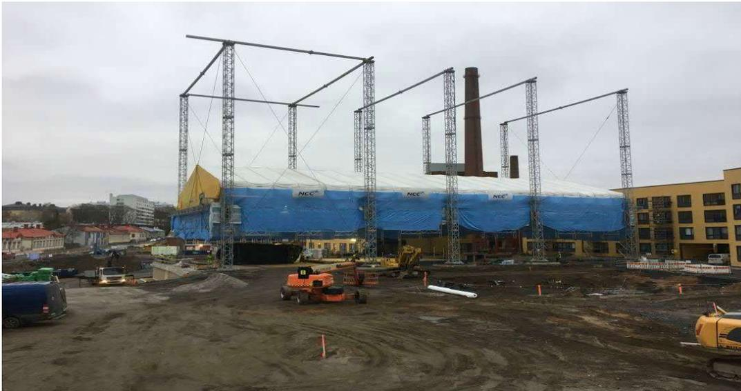
*Figure 1: Erection of weather protection for Puulinna.*
