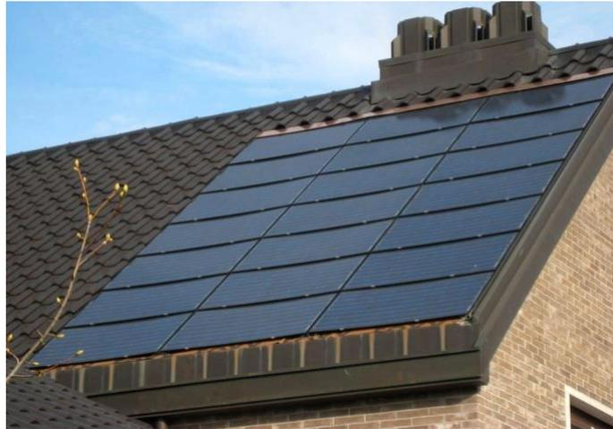
*Figure 3- Monocrystalline panels only taking up 50% of roof space while providing a sleek look*
