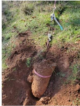
Figure 4. Removing existing concrete using a come-along
