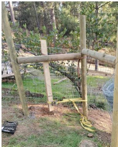
Figure 8. Fence tensioning with 2x4 clamp and ratchet straps
