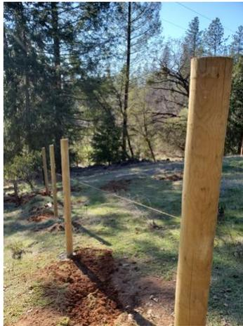
Figure 5. String line to ensure posts are placed flush to each other
