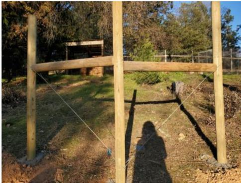
Figure 7. Corner H-bracing and cross brace wire
