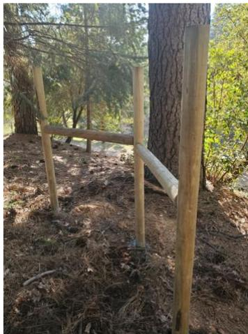
Figure 6. Corner H-bracing
