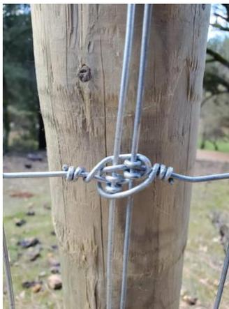
Figure 9. Fence splicing detail
