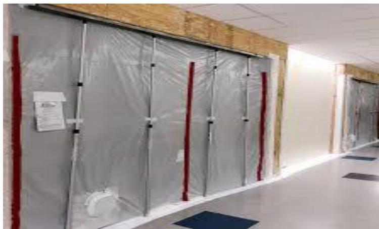
Figure 6. An example of a temporary zip wall.
