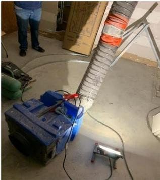
Figure 1. Negative air machine used on the project.
