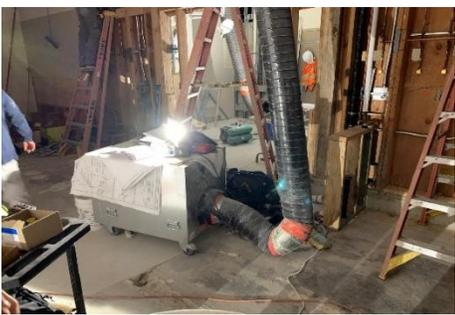
Figure 2. Negative air machine used on the project.
