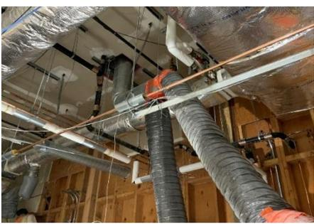
Figure 3. Shows how all negative air machines are connected and ejects air through the ceiling.
