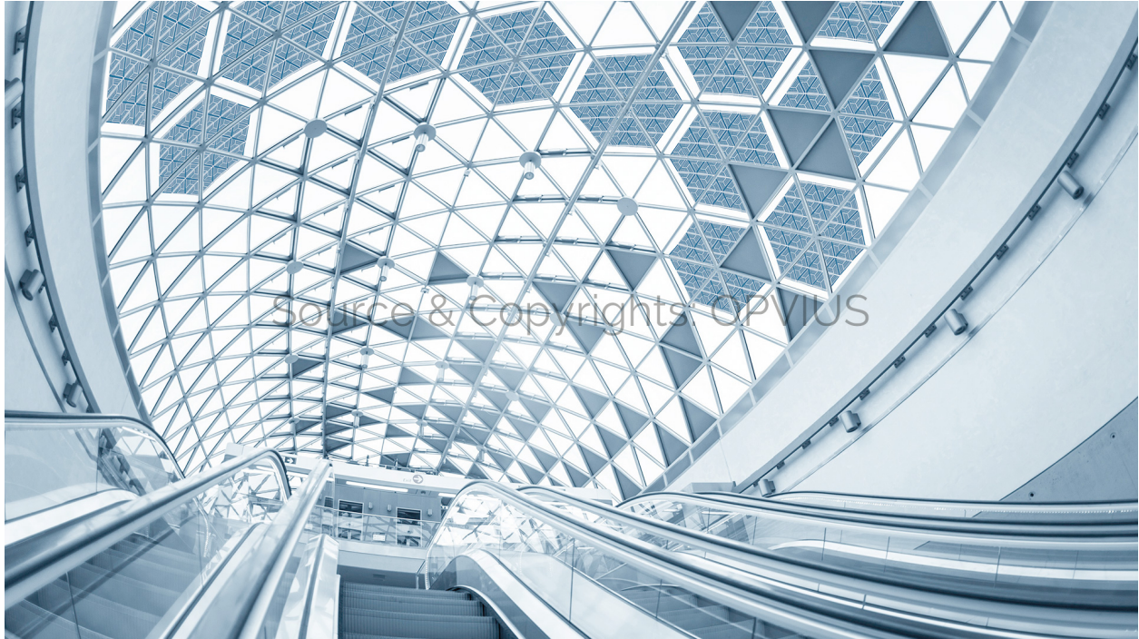
Figure 11: OPVIUS curved ceiling application[22]. Organic photovoltaic cells, due to their flexibility and easy to change design, can fit many different applications where inflexible (both mechanically and in design) inorganic photovoltaic panels will not. Image from © OPVIUS.
