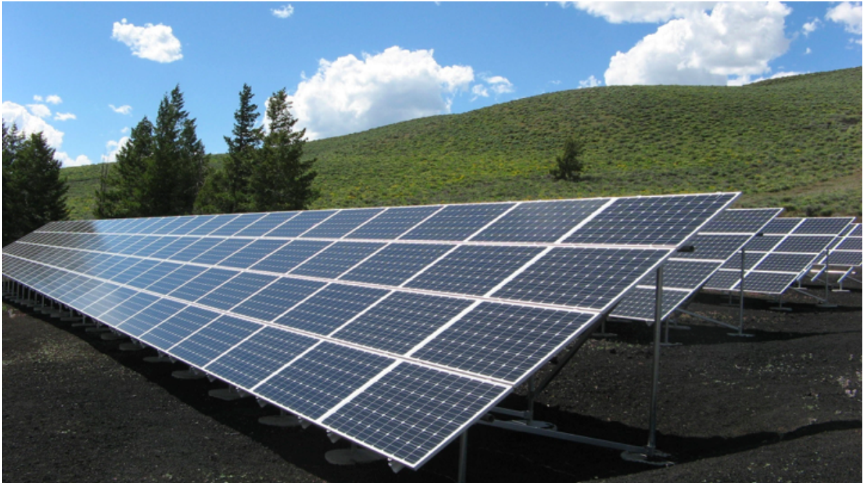
Figure 6 Mono-crystalline silicon photovoltaic array. Image released under CC0 (Creative Commons Zero). In areas clear of shading, large multiple acres of solar panels can generate several hundred megawatts to a couple gigawatts of power.
