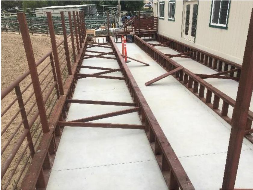
Figure C – Pony walls built with cross bracing installed
