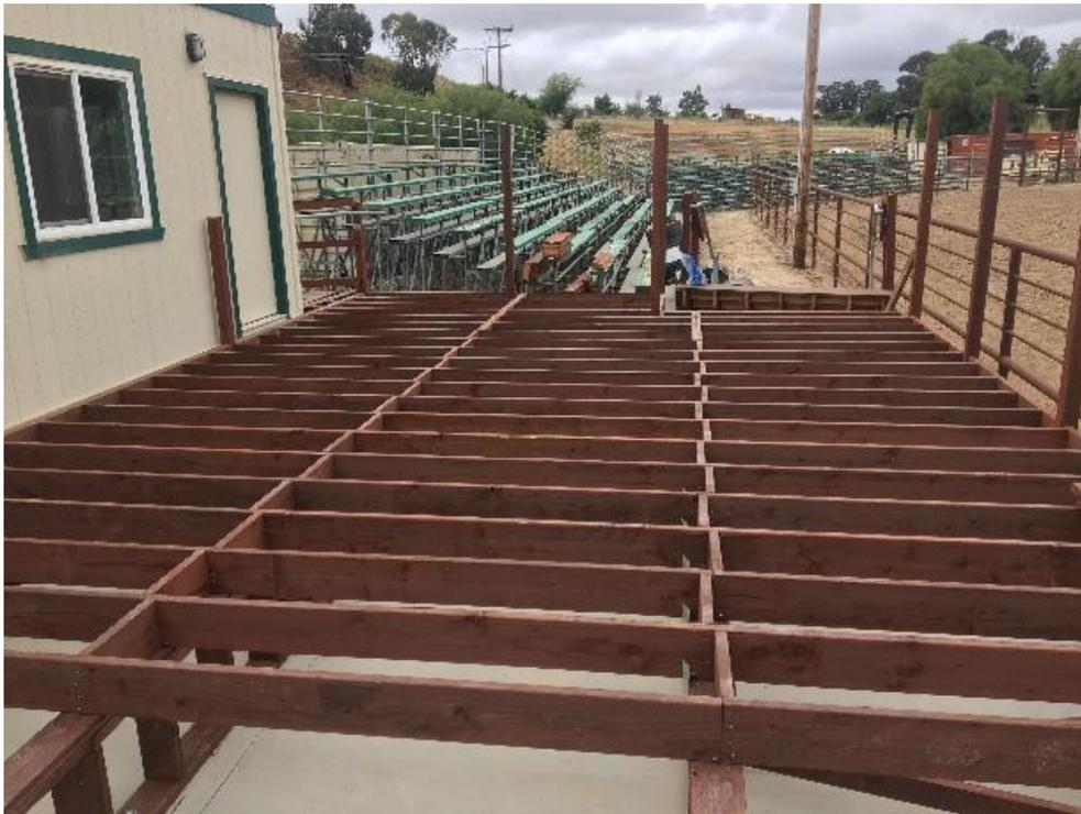
Figure D – Joists run over pony walls
