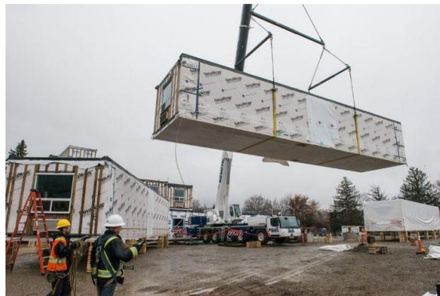
Figure 5- Module Being Lifted into Place On-site
