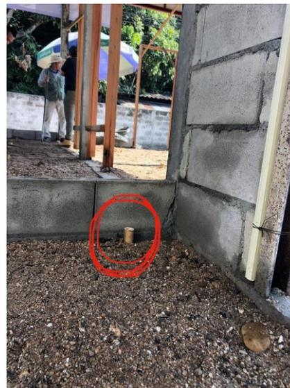
Figure 2b. Bamboo Stake Used to Signify Top of Slab for Slab on Grade Pour
