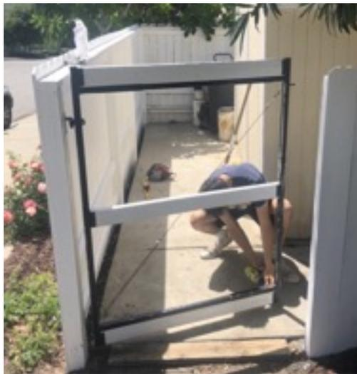
Figure 5. Gate frame with rails installed, no picket attachment yet
