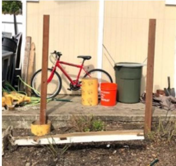
Figure 3. New posts set in concrete and completing leveling process
