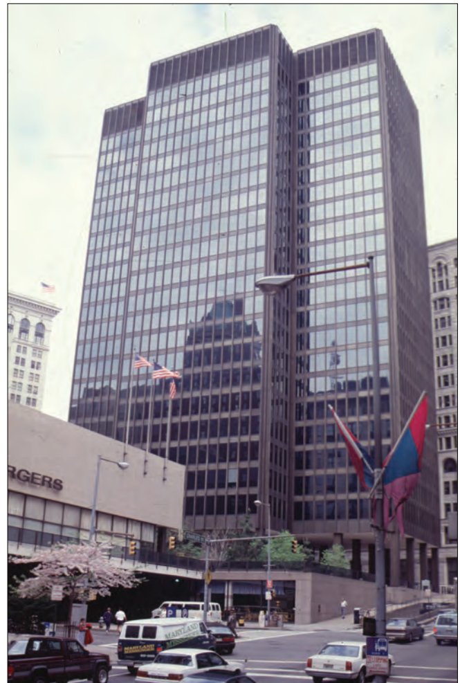
Figure 5: One Charles Center designed by Mies Van der Rohe, and the Hamburgers department store spanning over Fayette Street (demolished in the late 1980s). (photo by the author, 1985)
