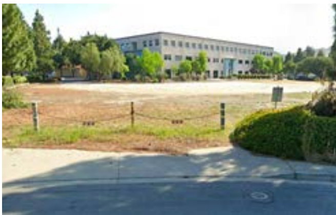
Figure 10: Street view of Site 5
