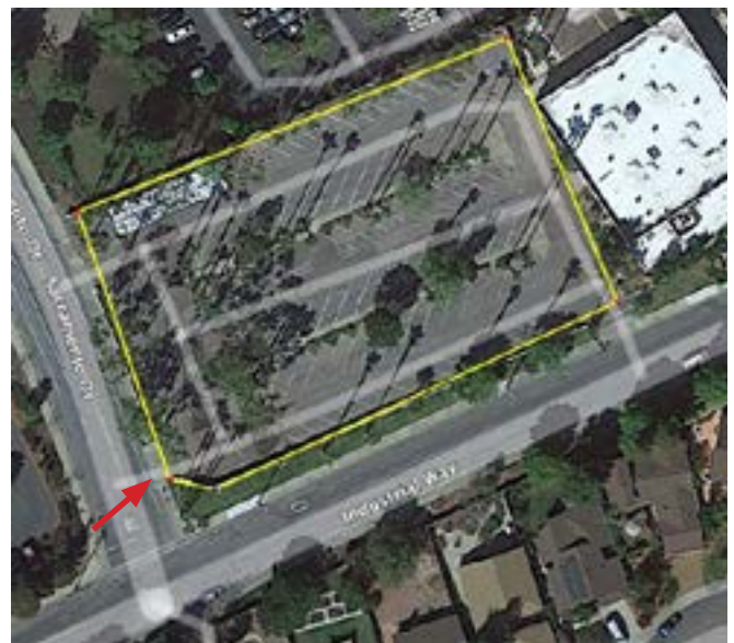
Figure 27: Aerial view of Site 13
