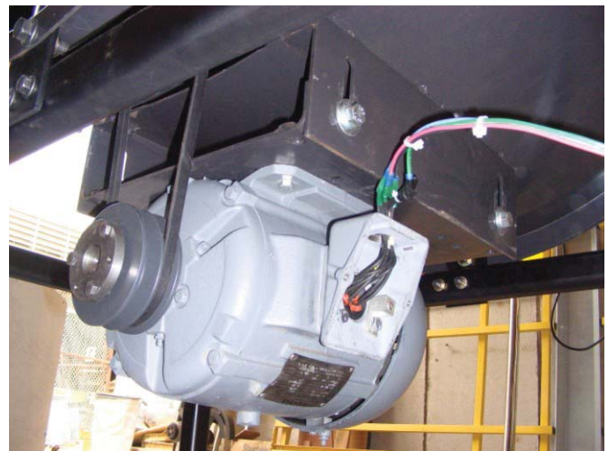
Figure 10. Installation of motor to the underside of fan.
