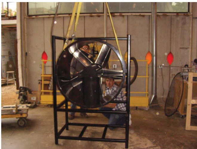
Figure 8. Installation of fan in motor stand.
