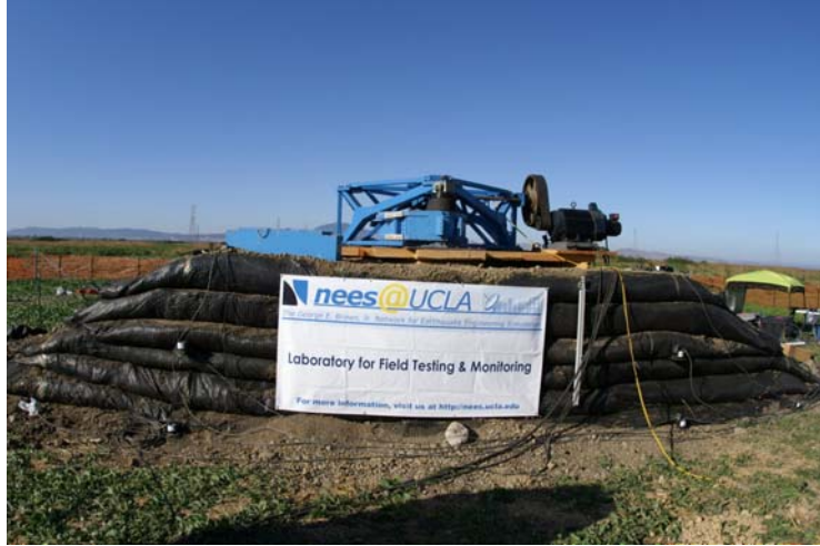
Figure 4. Photograph of the completed embankment with mounted MK-15 shaker.
