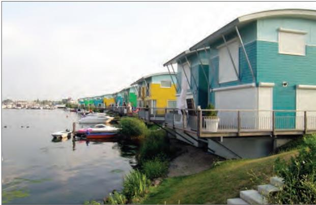
Figure 5: Netherland's Maas amphibious houses: located on firm soil, they are anchored to the site by a vertical structure and are prepared to float during a flood event. (photo: Factor Architecten and Dura Vermeer)
