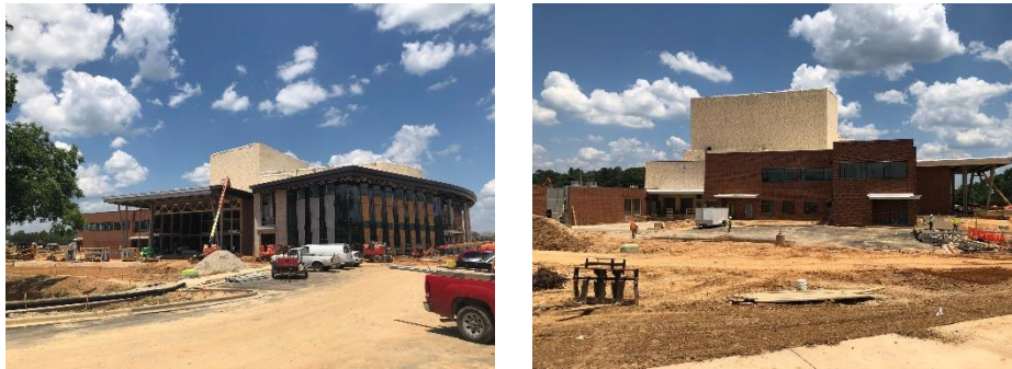
Figure 5: SAM100 completed work for the stage house (tallest portion of structure)
