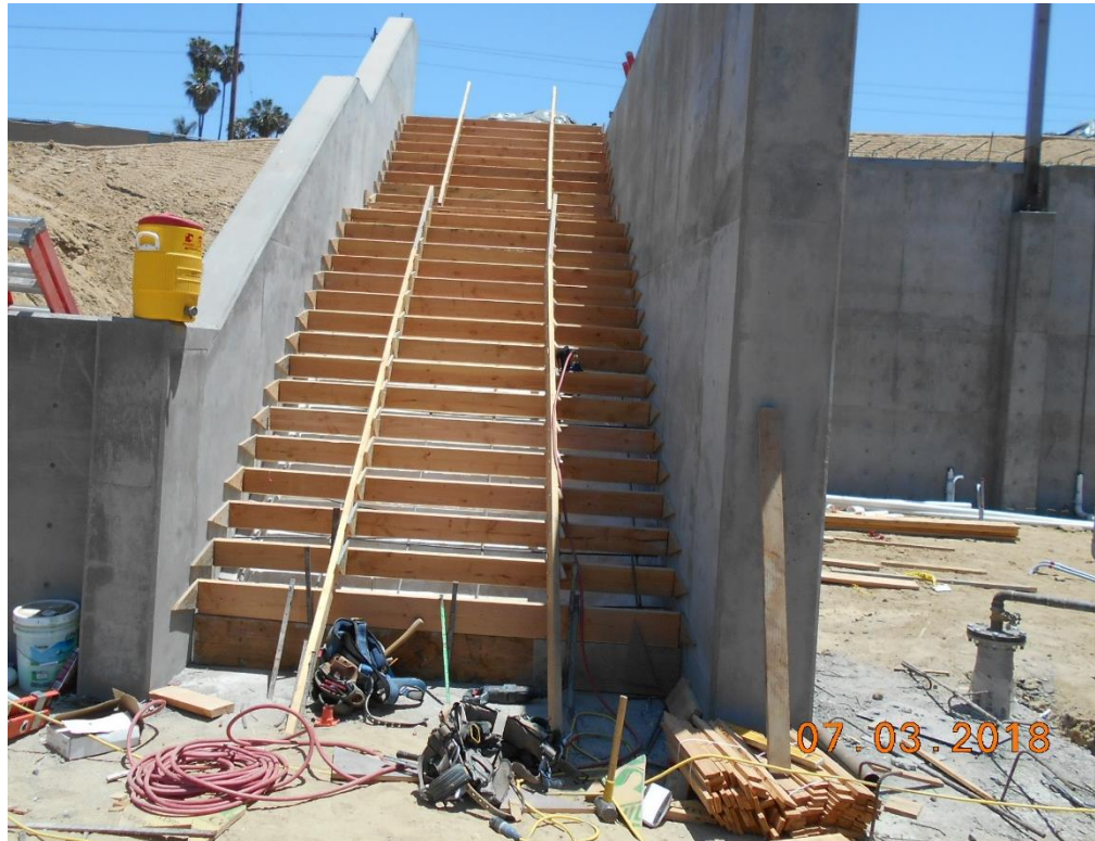
Figure 1: Location where Geofoam EPS 39 was installed Source: Courtesy of Superintendent
