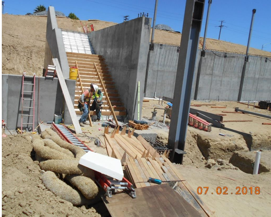
Figure 2: Location where Geofoam EPS 39 was installed
