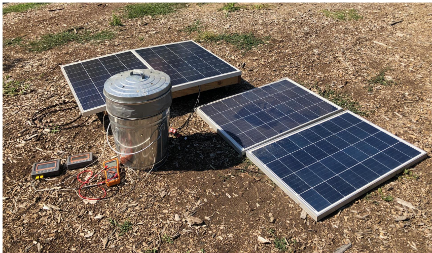
Fig. 7. Solar Salt ISECooker powered by four 100 W solar panels.
