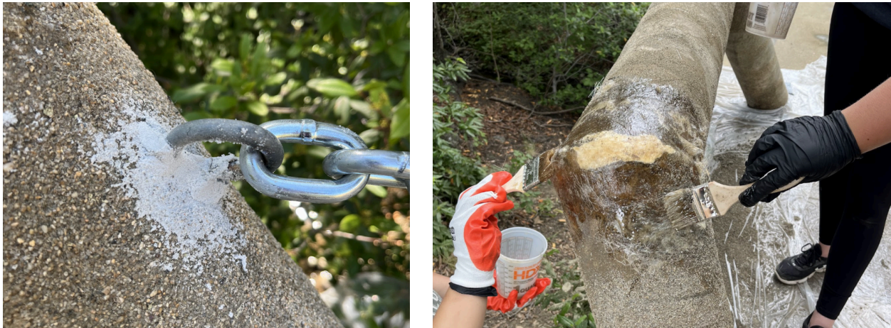
Figure 13 & 14: Grouted Hook & Fiberglass Over Filled Hole
