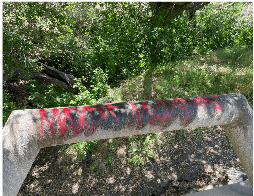
Figure 9: Graffiti Originally on Bridge
