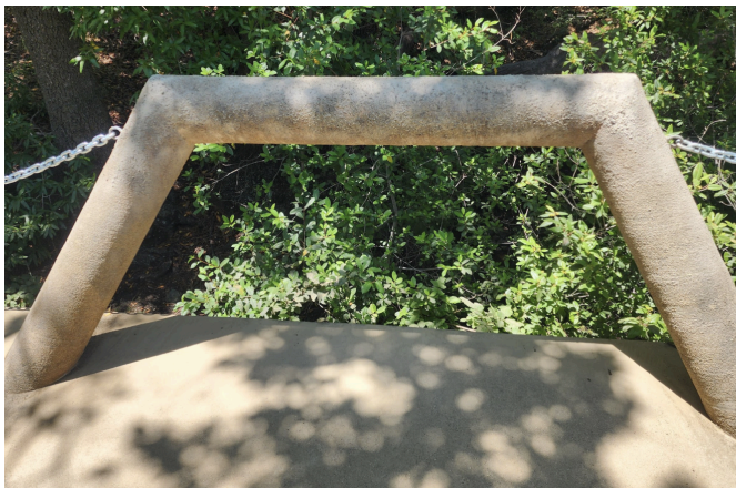
Figure 17: Restored Cylindrical Handrails
