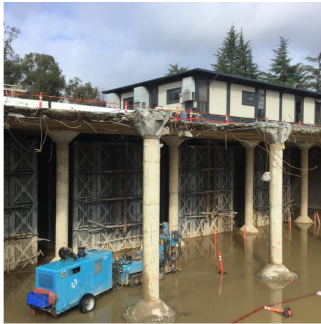
Figure 5: Photo of semi-excavated Ice Tank
