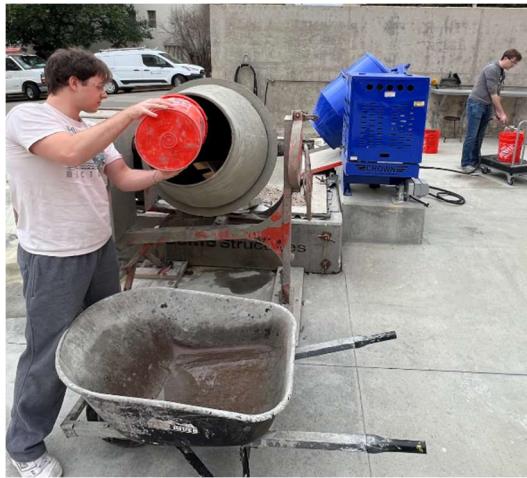
Figure 2 - CAED Concrete Yard
