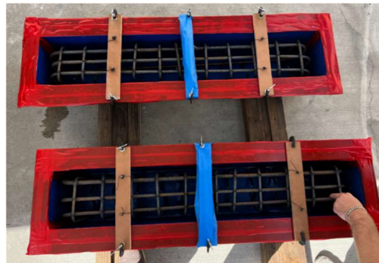
Figure 16 - Rebar Cage in Formwork
