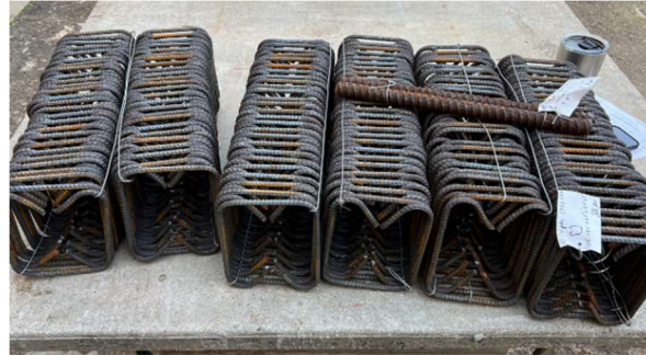
Figure 14 – Prefabricated Uniform Stirrups
