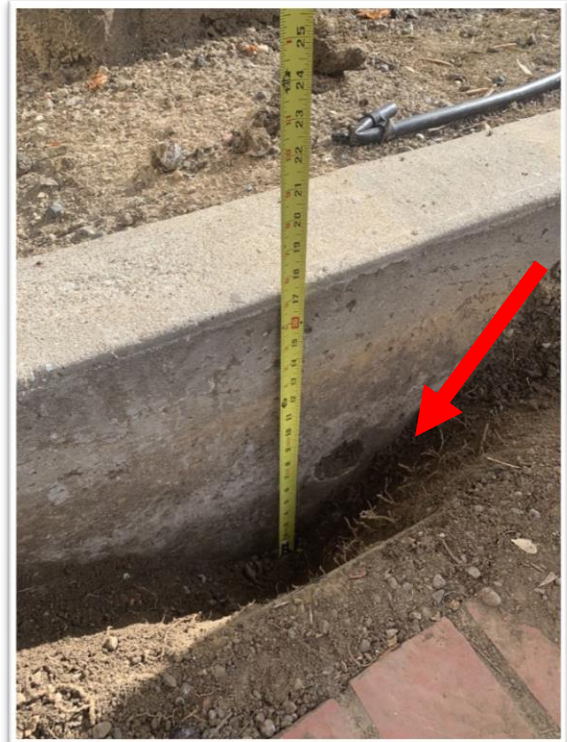
Fig. 3 Excavation of grade beam on existing structure
