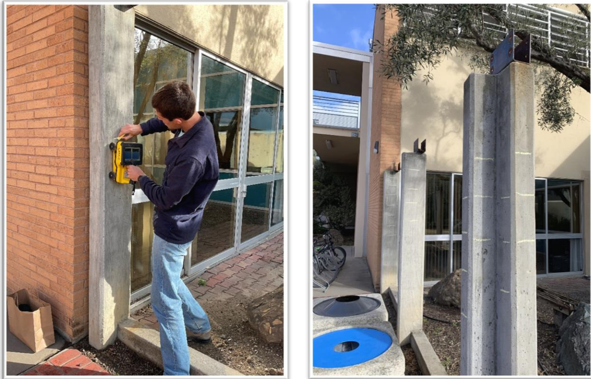
Fig. 6 Samuel Venable (Left) locating rebar in existing conditions with chalk
