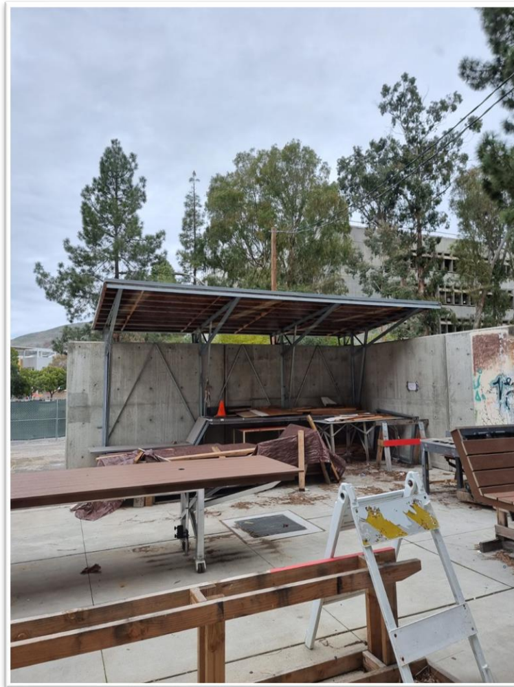
Fig. 9 Steel Canopy located near Architecture Bldg. 5
