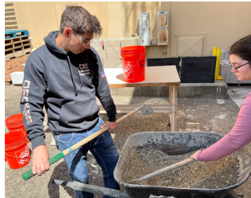
Figure 4. Mixing in wheelbarrow
