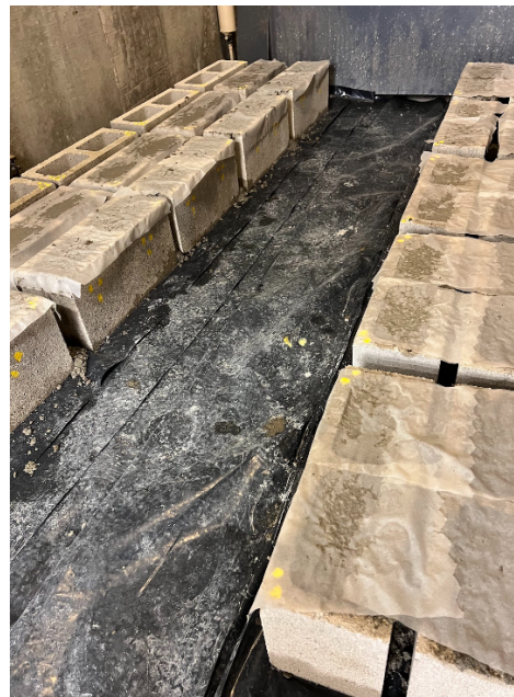
Figure 8. CMU blocks after filling cells and covering with damp cloth
