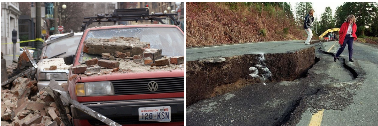
Figure 4.3: Damage after the 2001 Nisqually Earthquake [12,13]
