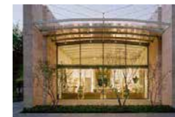
Close-up view of the north-west facade of the Nasher Sculpture Center. Image courtesy of Charles Sparks + Company. https://www.inexhibit.com/mymuseum/nasher-sculpture-center-dallas-texas/
