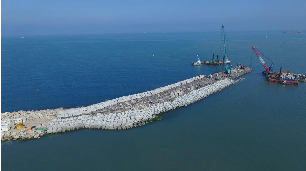
Figure 3 – New breakwater being constructed in Haifa, Israel
