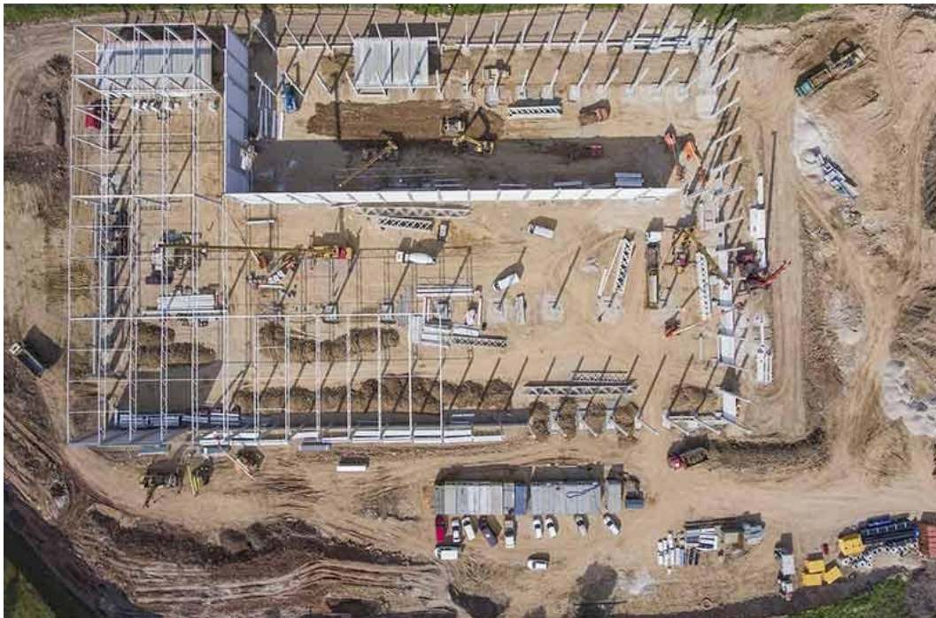
Figure 4 – Aerial view of construction site taken by drone
